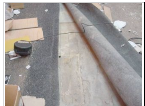
Concrete floor to centre
