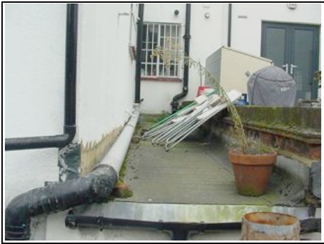
Flat roof over the shop
